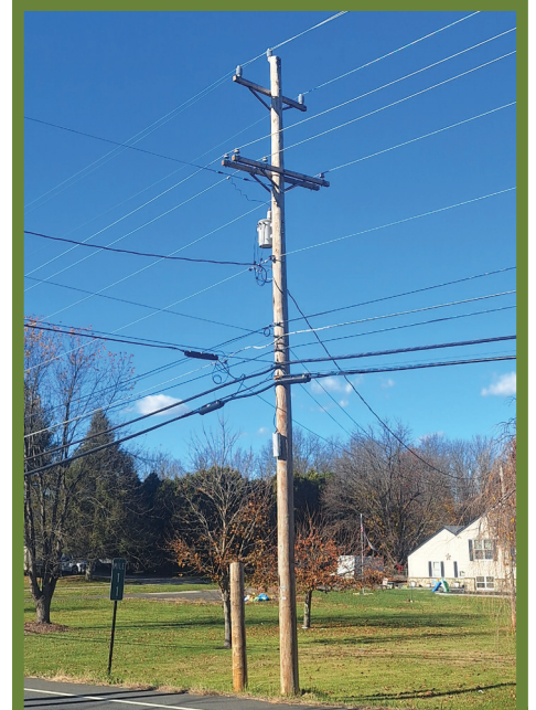
Pictured: An abandoned pole, shown to the left of the new pole. It has been cut short by the last company to transfer its wires to the new pole.
