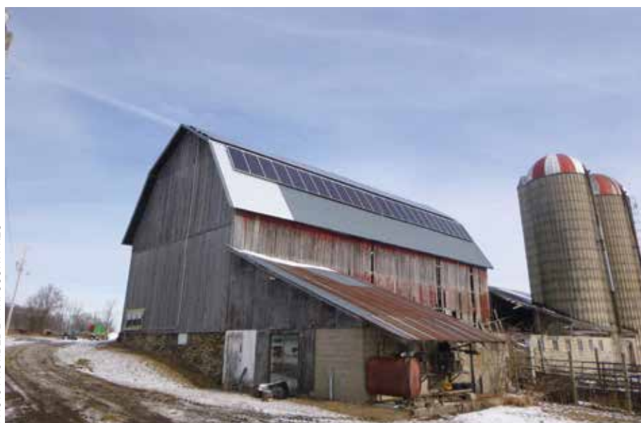
RENEWABLE ENERGY: The 600th consumer-owned renewable energy project interconnected with Pennsylvania-New Jersey cooperative lines is owned by Andrew Harding, Gillet, a member of Tri-County Rural Electric Cooperative. The 24.1-kilowatt solar system was put into service in February 2020. Currently, more than 700 consumer-member-owned renewable energy projects have been interconnected with cooperative lines in cooperation with Allegheny Electric Cooperative, Inc.
