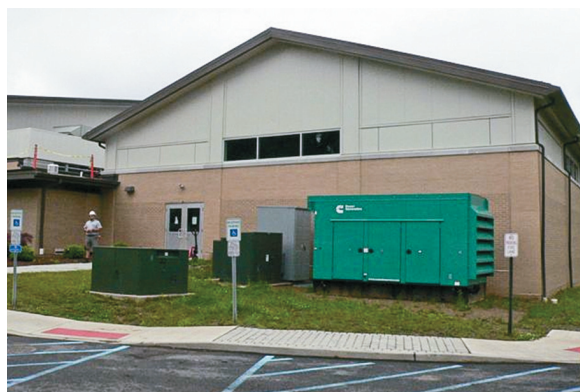
The DQDAA generator set installed beside the Centenary gym.
